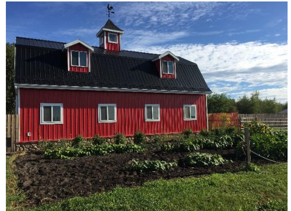
Our largest project so far, the construction of a gambrel roof barn, a heated winter home for the poultry flock.
